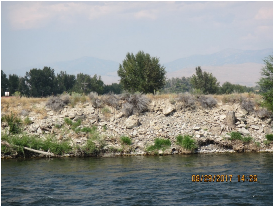
Figure 6. Damaged slope on downstream end
