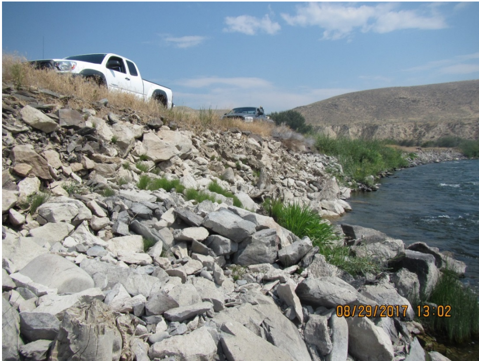
Figure 3. Damaged levee facing upstream
