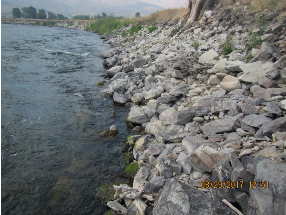
Figure 5. Eroded, over-steepened slope facing downstream
